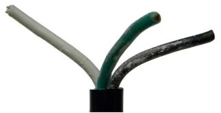
2. Next, strip the black wire and the white wire, giving yourself enough length to connect the ends to power. Depending on your application, you have the option to use quick connects or you can wire the fixtures in a more permanent method. Since this is a 12v system, a ground wire is not required, so you can trim the green wire flush to the sheath.
