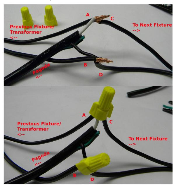
Repeat these steps for each of the fixtures and you'll have a permanent set of connections for your kit. After you test each of the lights in the run, apply silicone sealant inside each of the wire nuts to further protect the connections from the outside elements.
